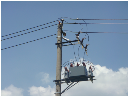
图 4 线路两组动态补偿安装实例 Fig.4 Instance of two groups of dynamic compensation installation on line
